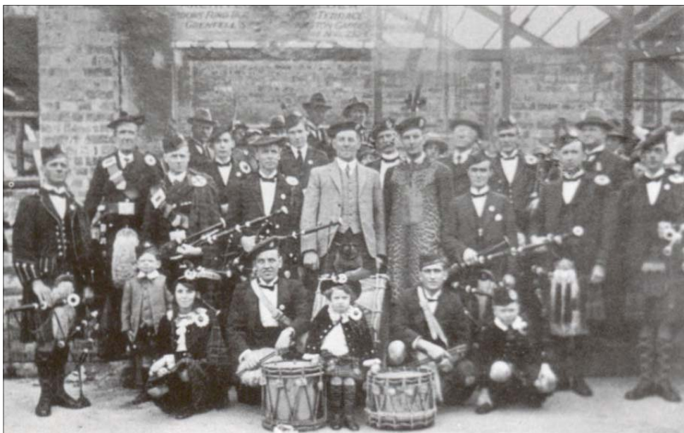
The Laying of the Foundation Stone of the New Building
